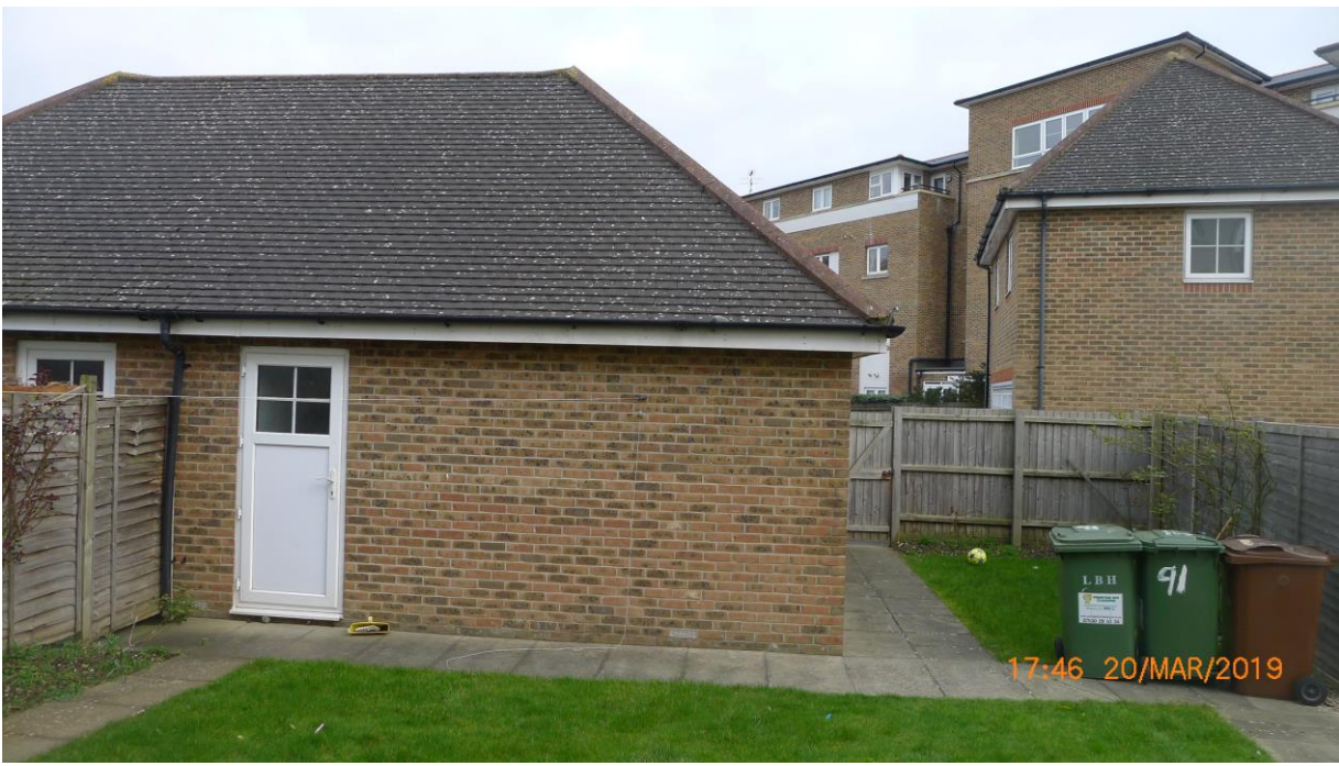
Above: Rear View towards Castlereagh House
